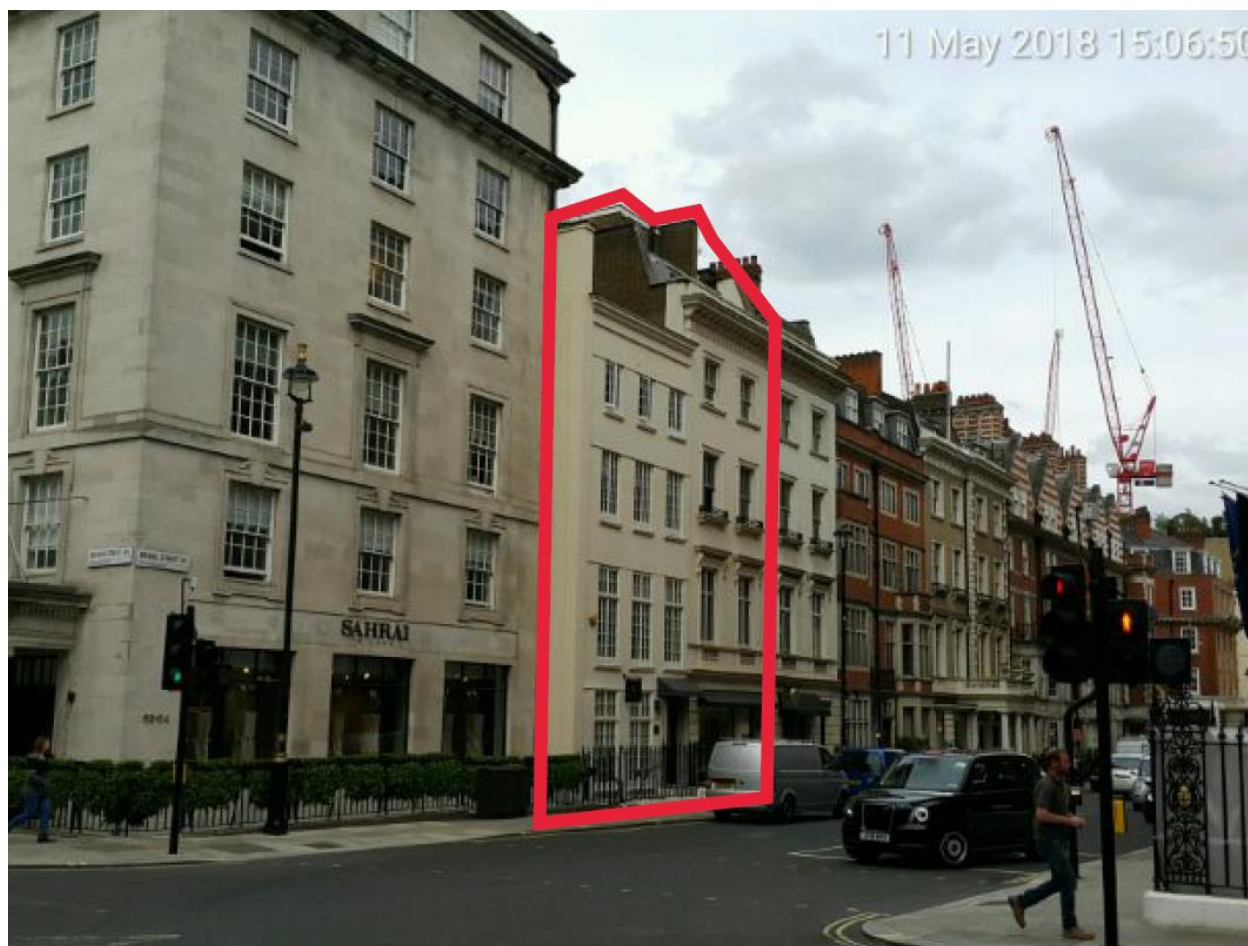
Sites 3 and 4 - 58 Brook Street (right) and 60 Brook Street (left).
